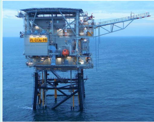
The PosHYdon pilot project is located at the offshore oil and gas platform off the coast of the Netherlands.
